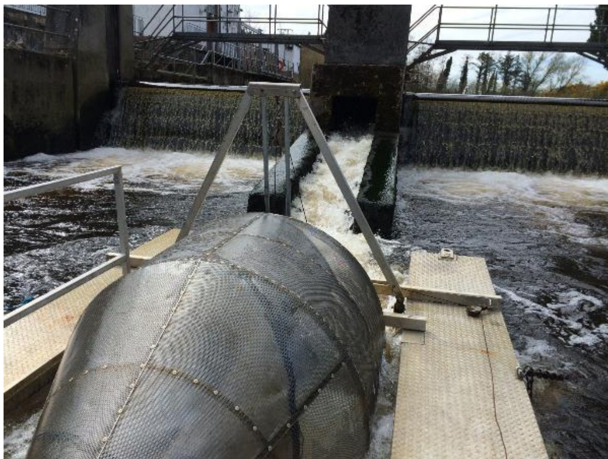
Fig 1. RST being hoisted into position at Campsie Barrage on the River Faughan, RST in fishing position in line with Denil fish pass.
